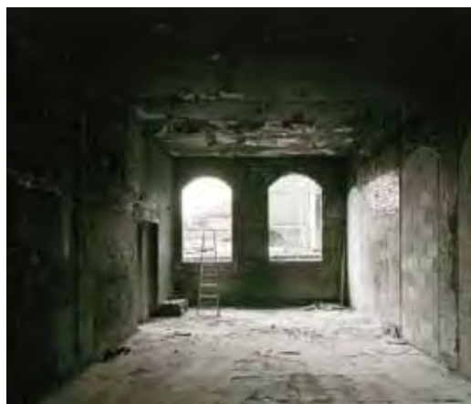
Interior of Fire Station pre-renovation Photos: John Riddy (1996)
