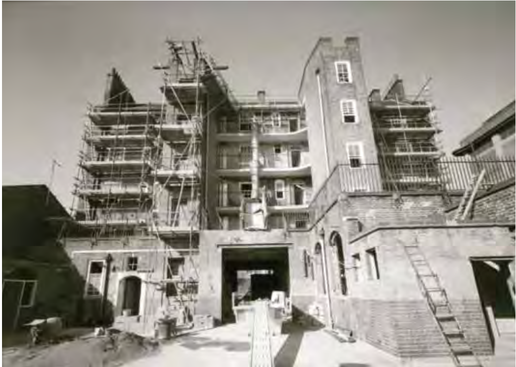
Exterior of Fire Station during renovation. Photo: John Riddy (1996)
