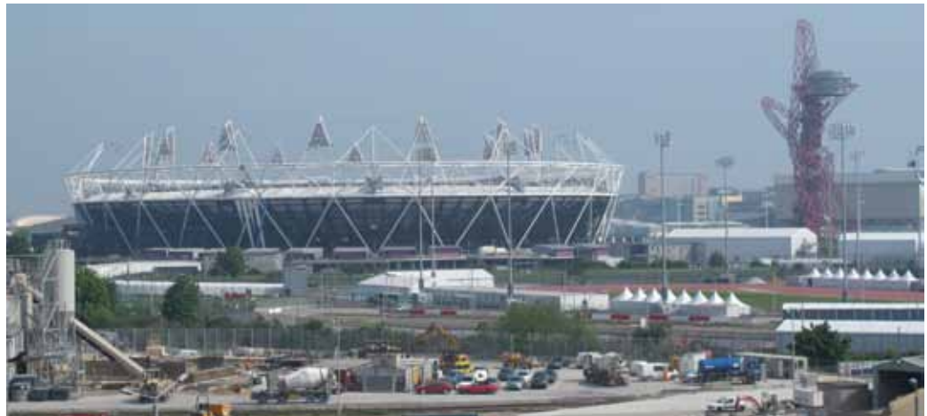
Olympic Stadium and Anish Kapoor's sculpture Orbit , under construction 2012
